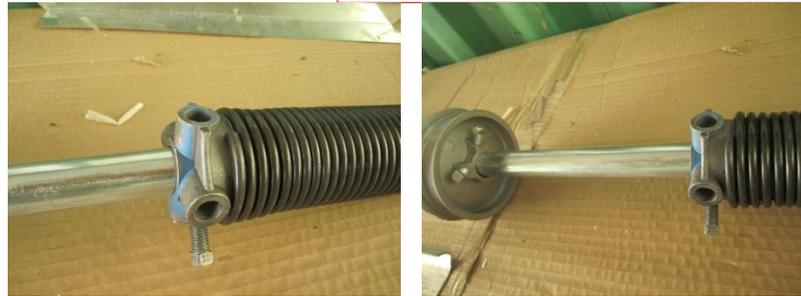
30. Place the shaft into the end bearing plates and once level use the lag bolts to secure the center bearing plate to the header.
