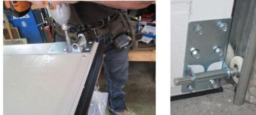
10. Install the side brackets at the top of the panel with the small hinge upwards. See illustration.
