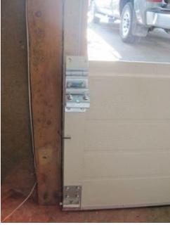
14. Insert the rollers into the appropriate locations in the bottom and end hinges. Hang the cables over the top roller.
