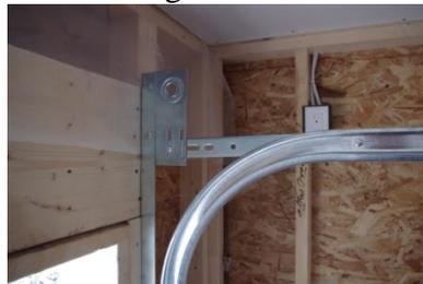
25. Attach the horizontal track (curved) to the vertical track at the flag bracket.
