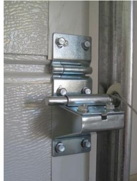
11. Measure the location for the center hinge(s). One for the 9' wide panel and three for the 16' wide panel. (Middle of panel for 9' panel and every 48" for the 16' panel). Note: The center hinges are to be installed with the small side down and the large side up.
