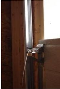
15. Take another panel and install the side brackets at the top of the panel with the small hinge upwards similar to step 9.
