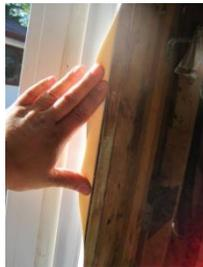
6. Measure cut and install the side weather-strips using pan head screws. Pre-drill the holes approximately 8" apart for the screws.
