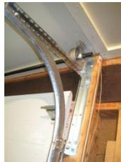
31. Secure the springs to the center bearing plate using the largest bolts provided.
